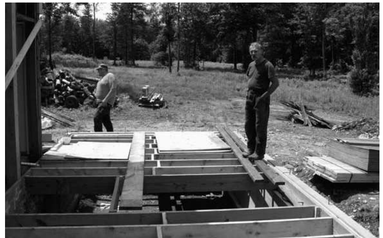
Gary Forish and Mark Bidus work on the North Cottage.
