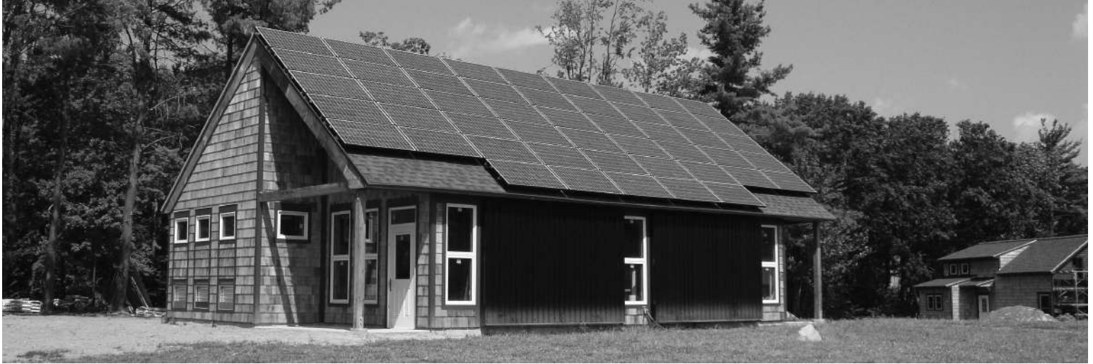
At Noble View Outdoor Center, the bathhouse's exterior is completed. It's expected to be open this November. photo by Gary Forish
