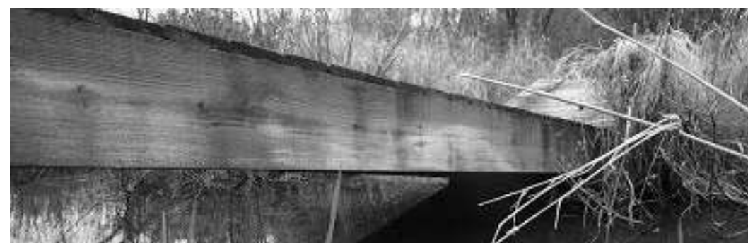
Above: Hubbard Brook Boardwalk Before
