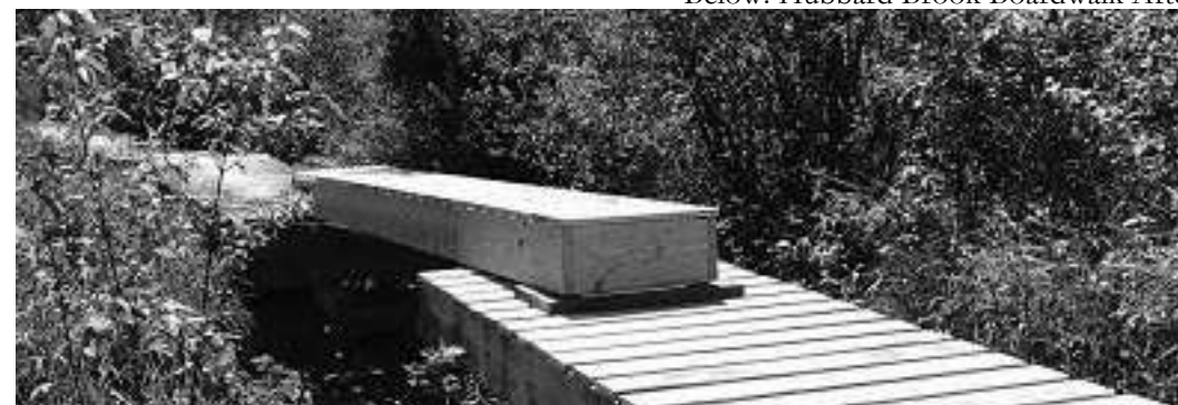
Below: Hubbard Brook Boardwalk After
